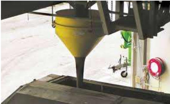
Sustainable Operation – No electricity required
